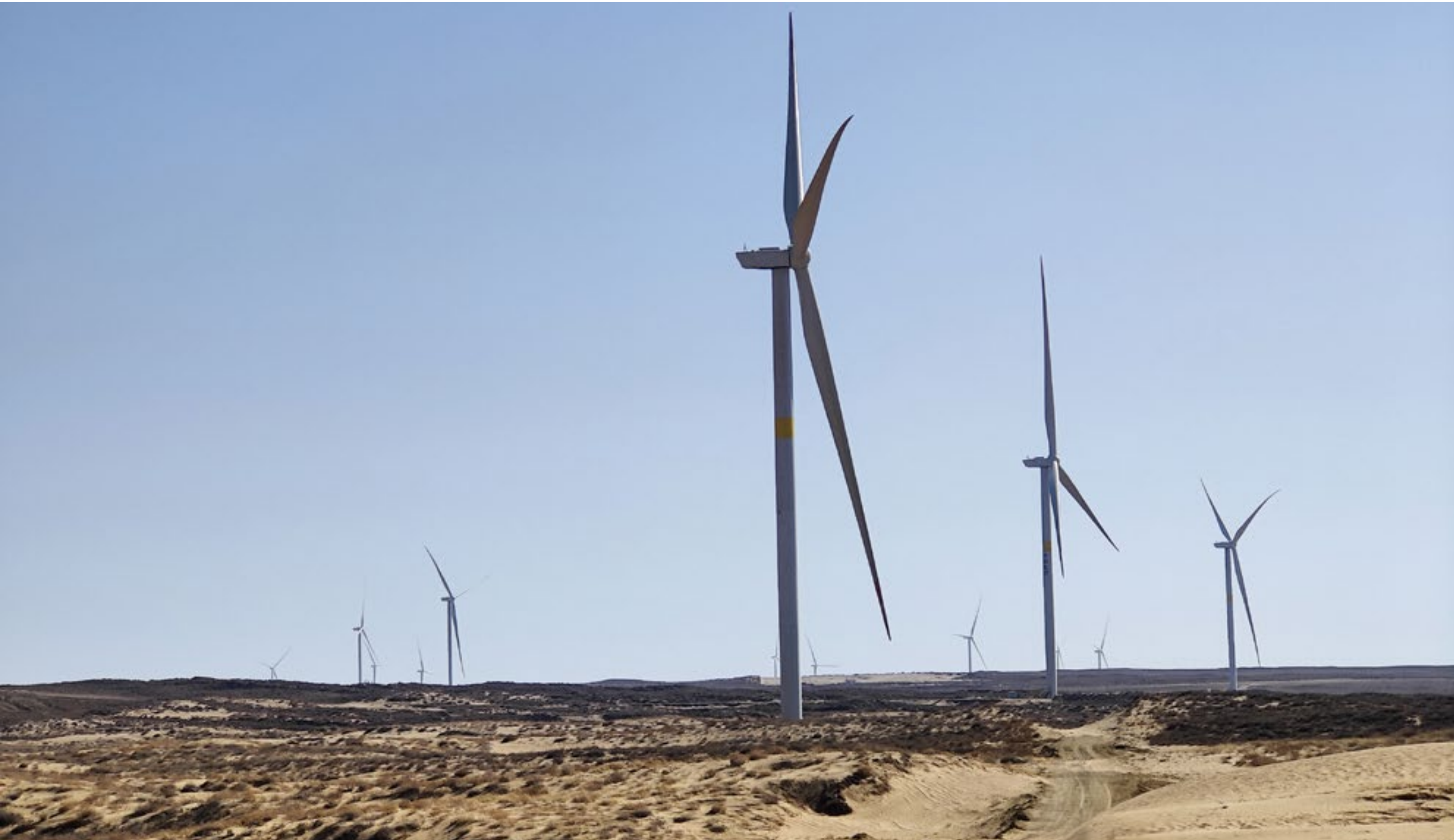
Pilot commissioning of Wind EBF in Inner Mongolia
